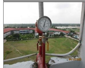
External photo(s) of the production unit(s) Water pressure of fire hose pipe.JPG
