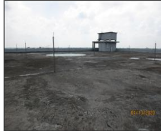
External photo(s) of the production unit(s) Rooftop.JPG
